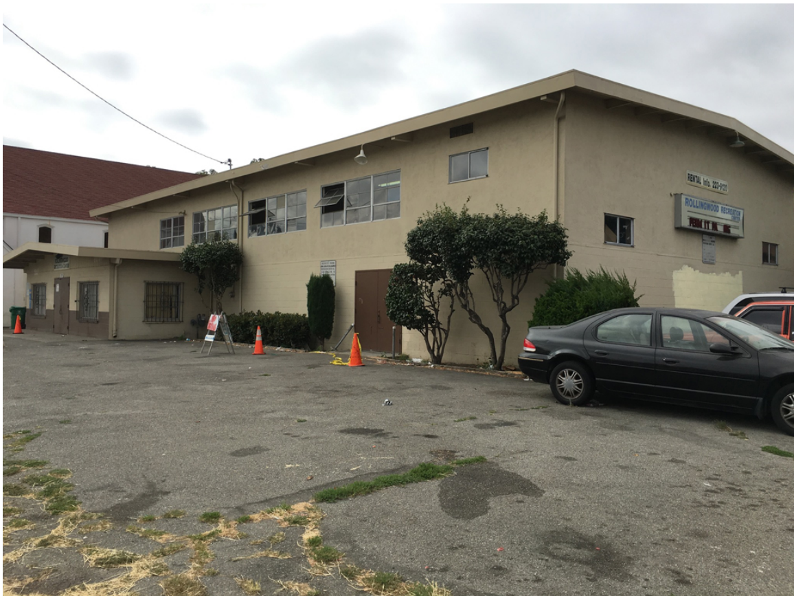
Figure 3 Exterior of RWPRD Facility
